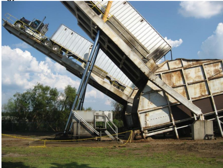
Figure A1: The chip dump at Craven Wood Energy, New Burn, NC
